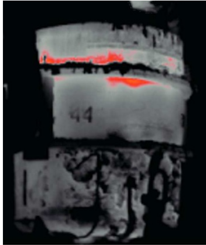
Alarm colors highlight potentially problematic areas in the thermal images
